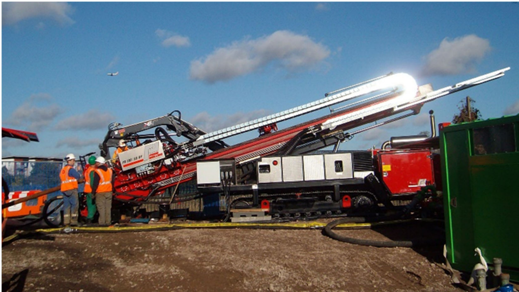
Figure 7: Photo of Typical Horizontal Directional Drilling Rig
